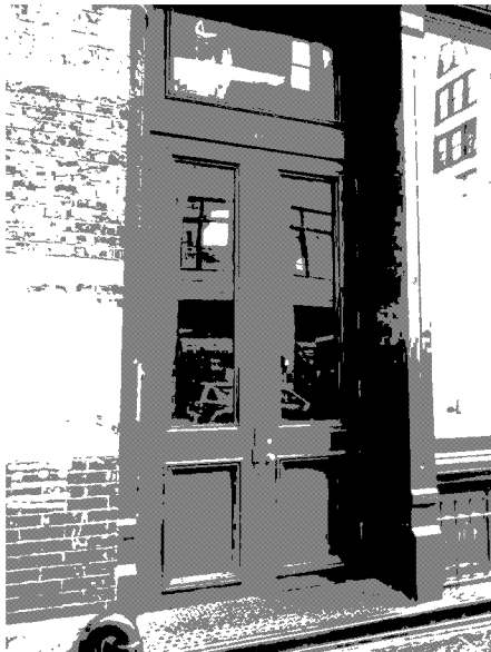
SUBJECT UNIT #2B'S ENTRANCE TO THE BUILDING
