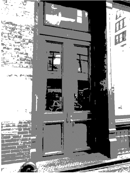
SUBJECT UNIT #2B'S ENTRANCE TO THE BUILDING
